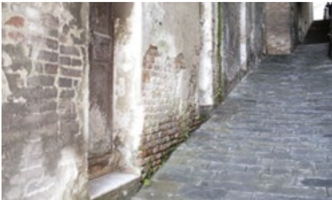
Destruction of render and mortar joints
