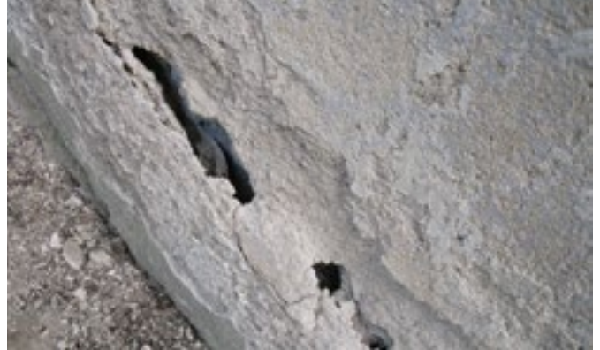
Damaged plaster
